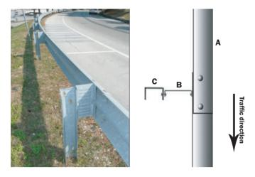
FIG. 1—Guardrail: photograph and schematic view from above.  $A = beam; B = distancer; C = \Box$ -shaped post.
